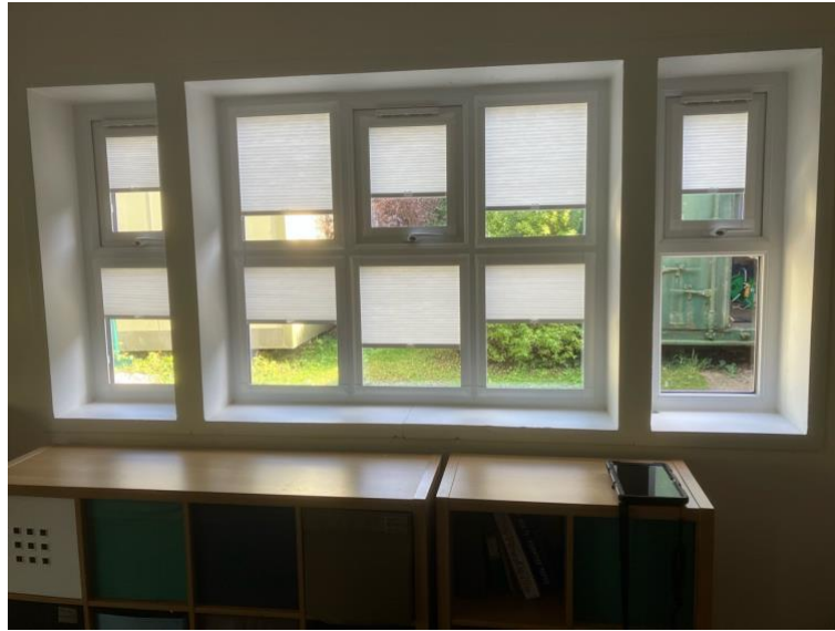
Image 14: New windows at Bedminster Quakers Meeting House
